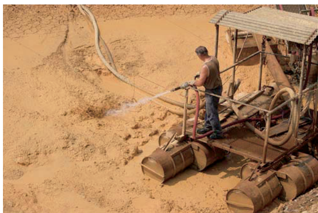
Cleaning of one of the three settlement ponds for active mine water treatment of the abandoned Straßberg/Harz fluorite mine.
